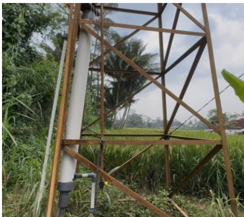
Gambar 7 Tabung Filter Multi Media
